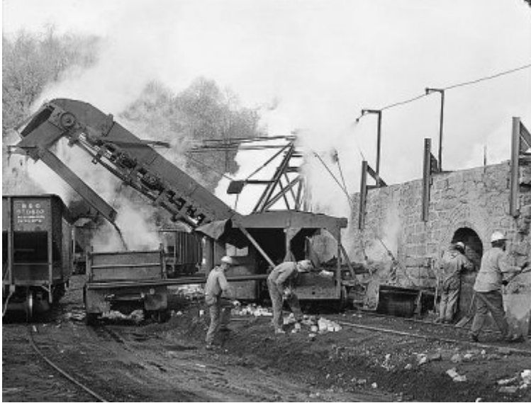
Here is a picture from 1974 of the extractor pulling coke from an oven and loading it into rail cars. A flume on the machine catches the "dribble." (Public domain photo by William Barrett, HAER (Historical American Engineering Record))
